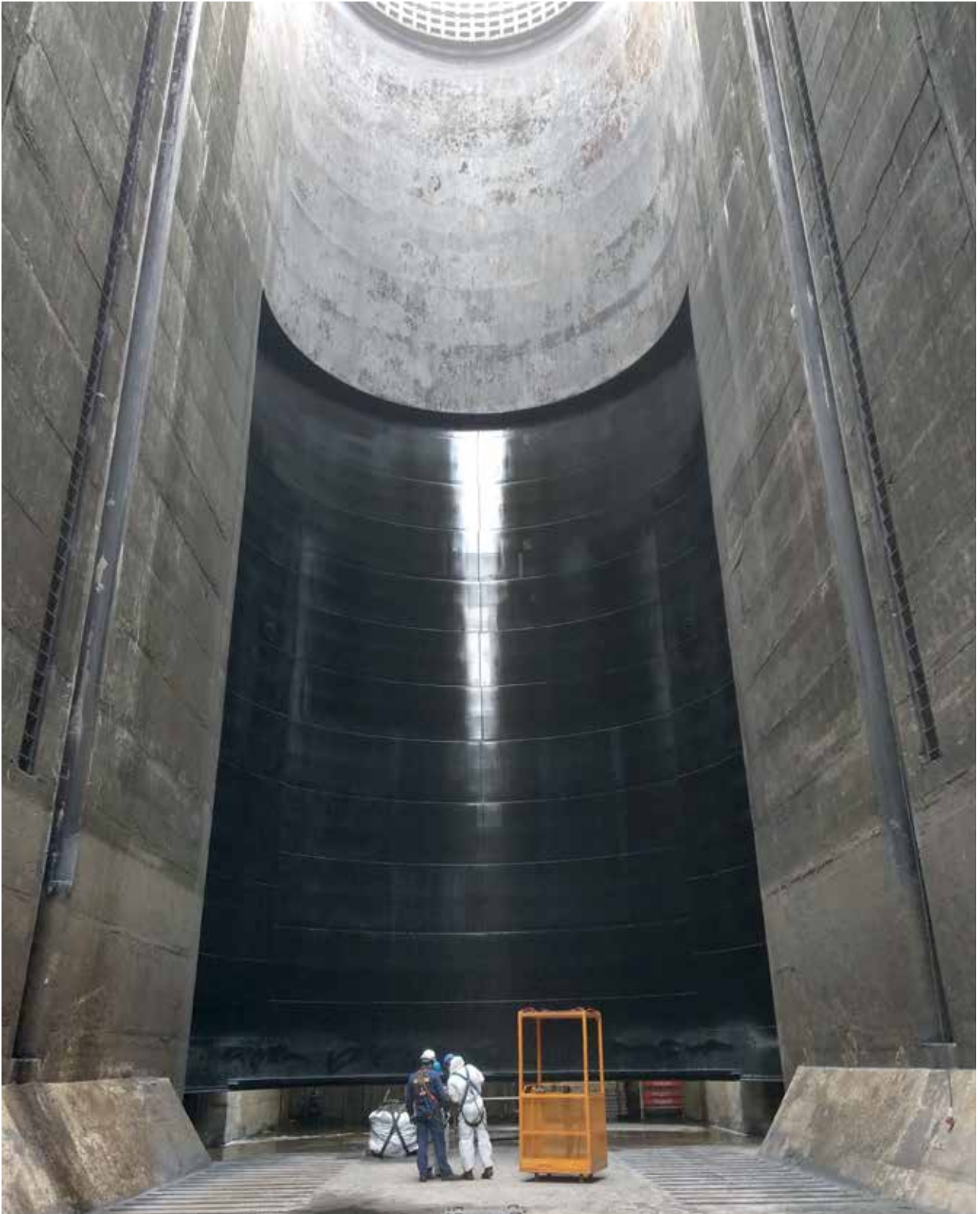
EDP - Carrapatelo Power Plant - Improvement of Navigation Lock Equipment CARRAPATELO - PORTUGAL
