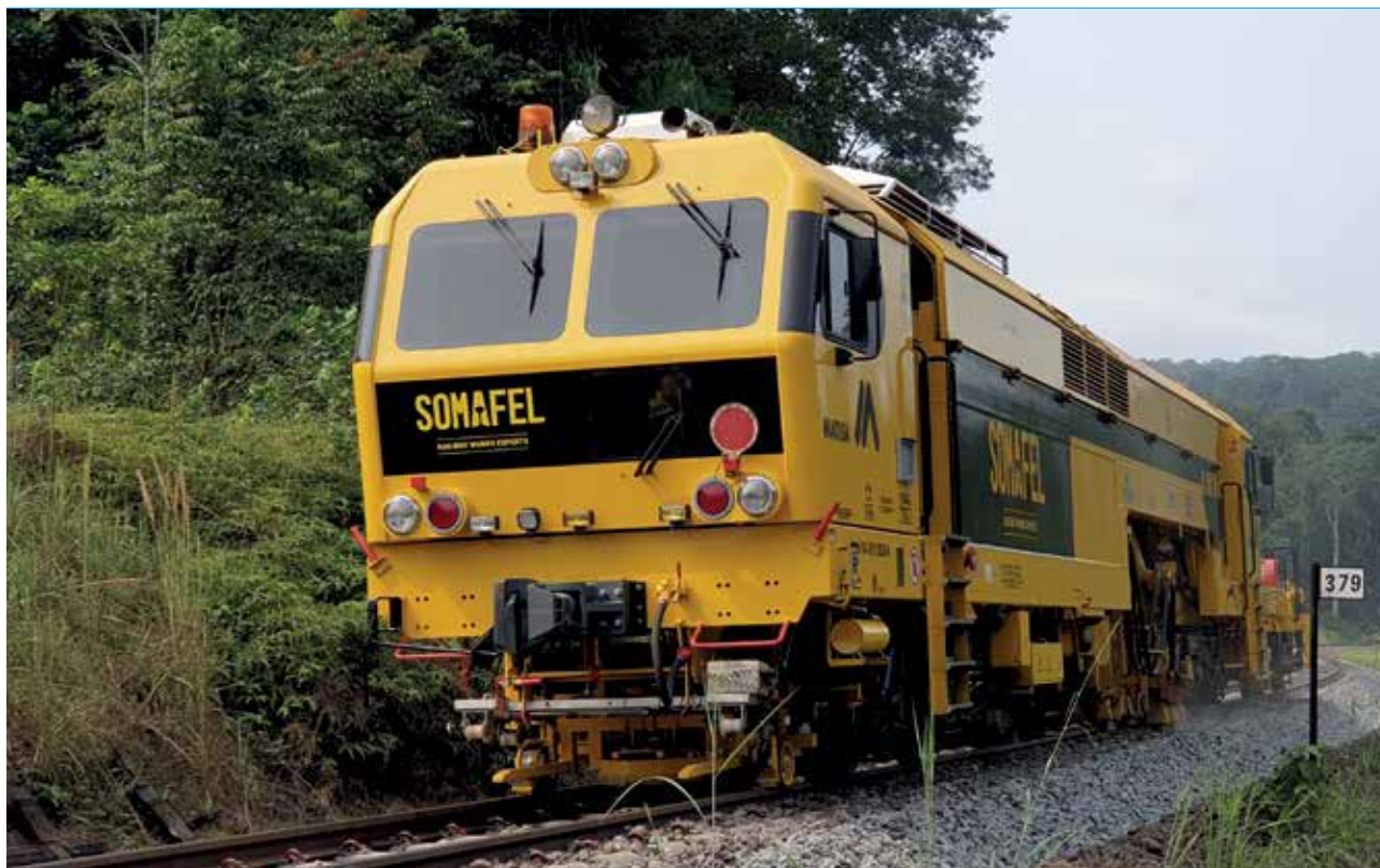
SETRAG - Ballast regularization work and heavy mechanical tamping of the Trans-Gabon railway GABON
