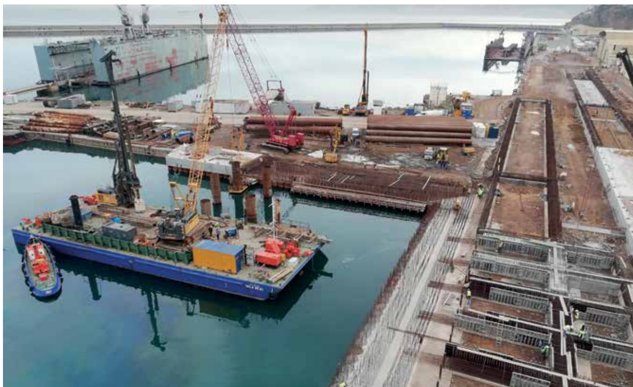
ECRN - Construction of a Ship Lift with a Lifting Capacity of 9,000 tonnes or more MERS EL KÉBIR NAVAL BASE - ALGERIA
