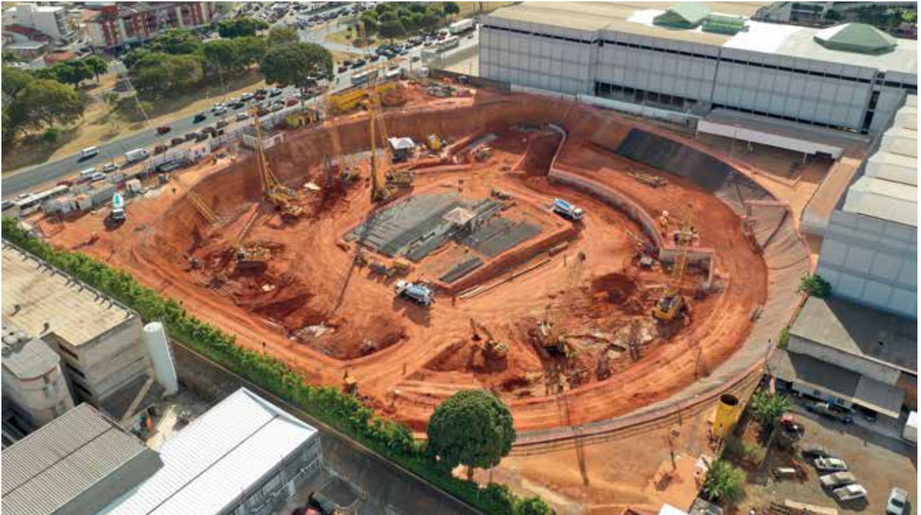
Execution of Excavations, Partial Foundations and Peripheral Containment for the IURD Cathedral BRASILIA - BRAZIL
