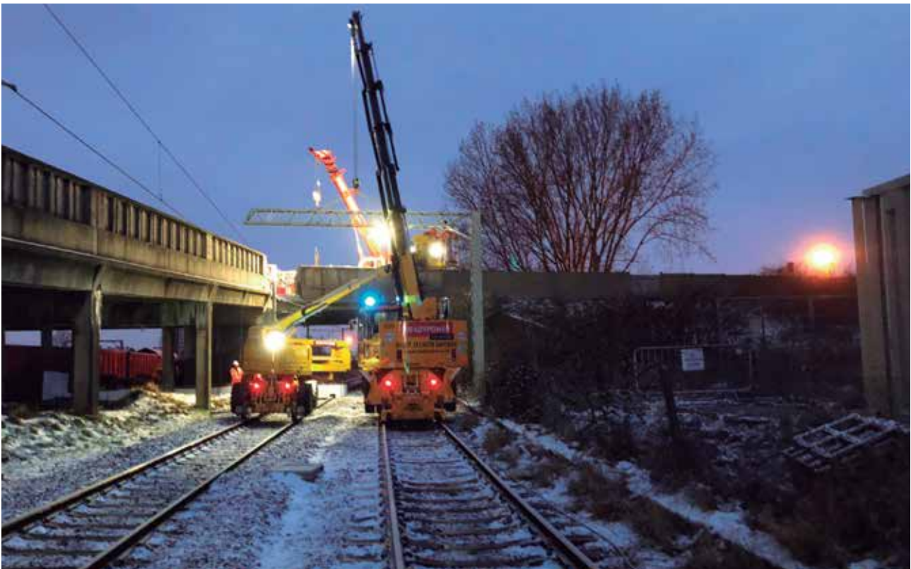
Crossrail South East Section Project BARKING RIVERSIDE EXTENSION - ANGLETERRE
