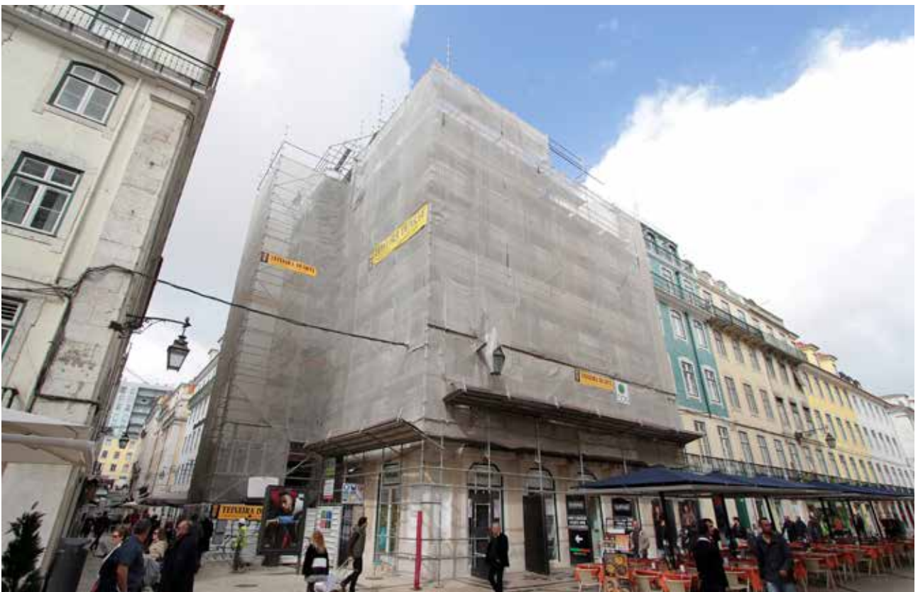
HOSTELING YOU - EDIFICIO MY STORY HOTEL AUGUSTA Lisboa - Portugal
