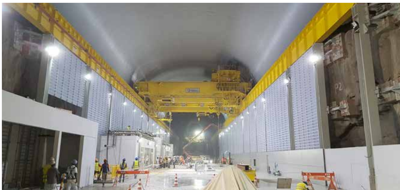
NORBERTO ODEBRECHT CONSTRUCTION COMPANY - LAÚCA HYDROELECTRIC POWER STATION - ASSEMBLY OF METAL STRUCTURES FOR THE POWER HOUSE Laúca - Angola
