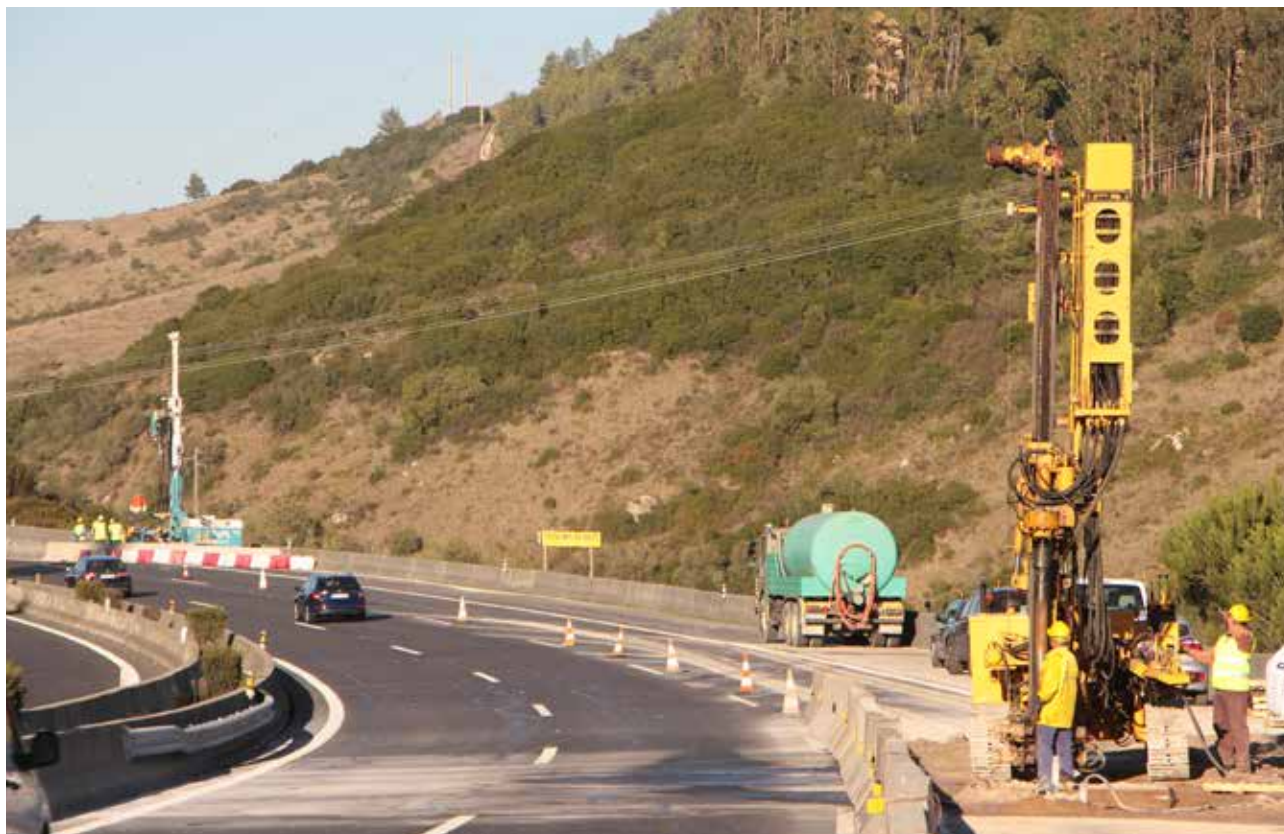
BRISA CONSOLIDATION OF LANDFILL KM 25+700 OF THE A9 - CREL - CONSOLIDATION INJECTIONS São Julião Do Tojal - Portugal
