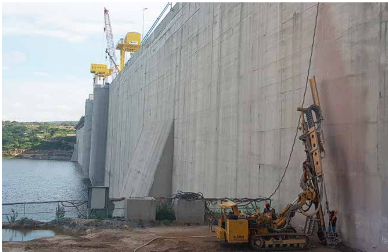
NORBERTO ODEBRECHT CONSTRUCTION COMPANY - A.H. LAUCA PROJECT - PROVISION OF DRILLING, WATERPROOFING INJECTION AND BORING FOR DRAINAGE SERVICES Angola
