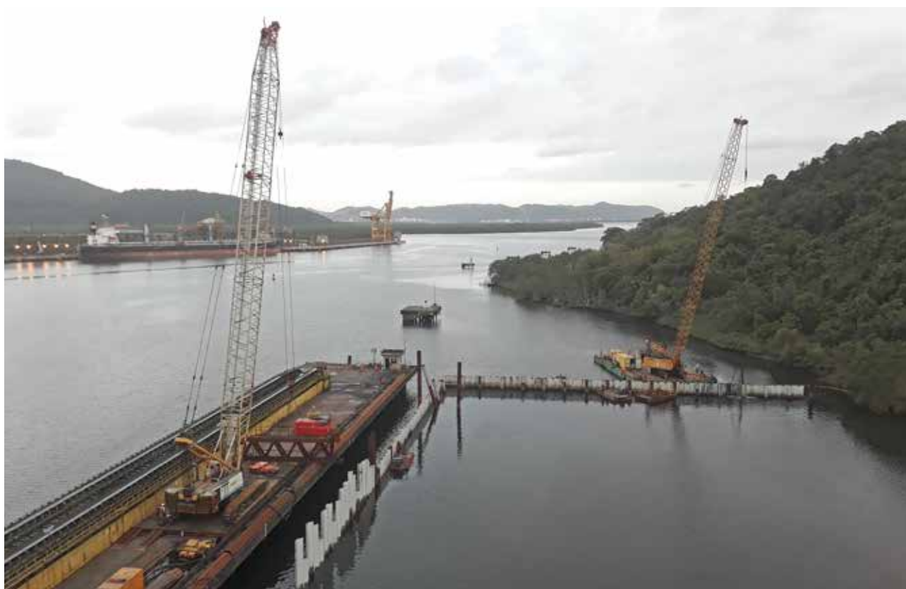
VLI - SHEET PILING CONTAINMENT - PIAÇAGUERA CHANNEL Cubatão - Brazil
