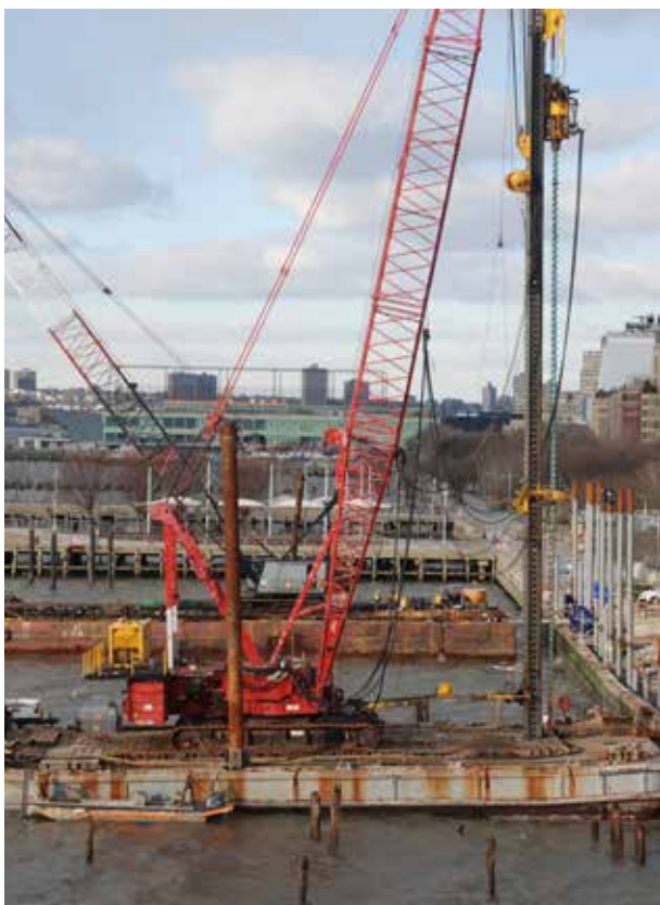
NYC EDC & SKANSKA USA BUILDING INC - INSTALLATION OF FLOATING QUAYS FOR FERRY BOATS - EXECUTION OF METAL PILINGS - RIO HUDSON New York - USA
