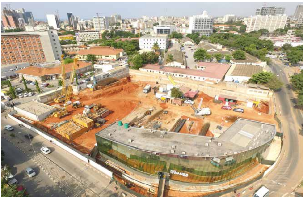
AFRIQUE IMO CORPORATION EXCAVATION AND PERIPHERAL RETENTION Luanda - Angola
