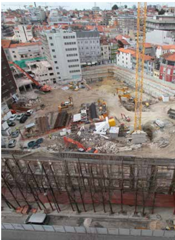
INTERFUNDOS - D. JOÃO I NEIGHBORHOOD - DEMOLITION, FAÇADE CONTAINMENT, EXCAVATION AND PERIPHERAL CONTAINMENT Porto - Portugal
