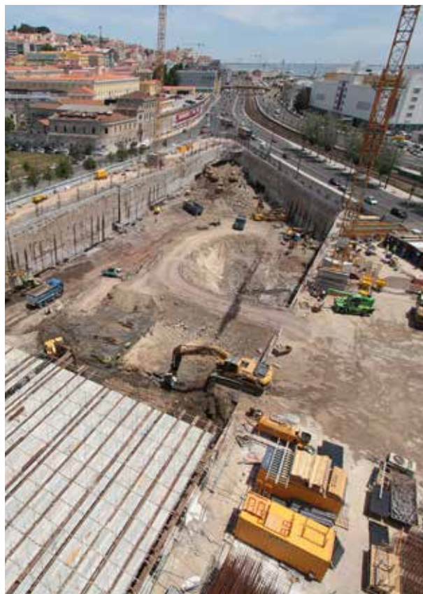
IMO HEALTH - EXCAVATION, PERIPHERAL CONTAINMENT AND FLOOR 0 STRUCTURE - CUF TEJO HOSPITAL Lisbon - Portugal
