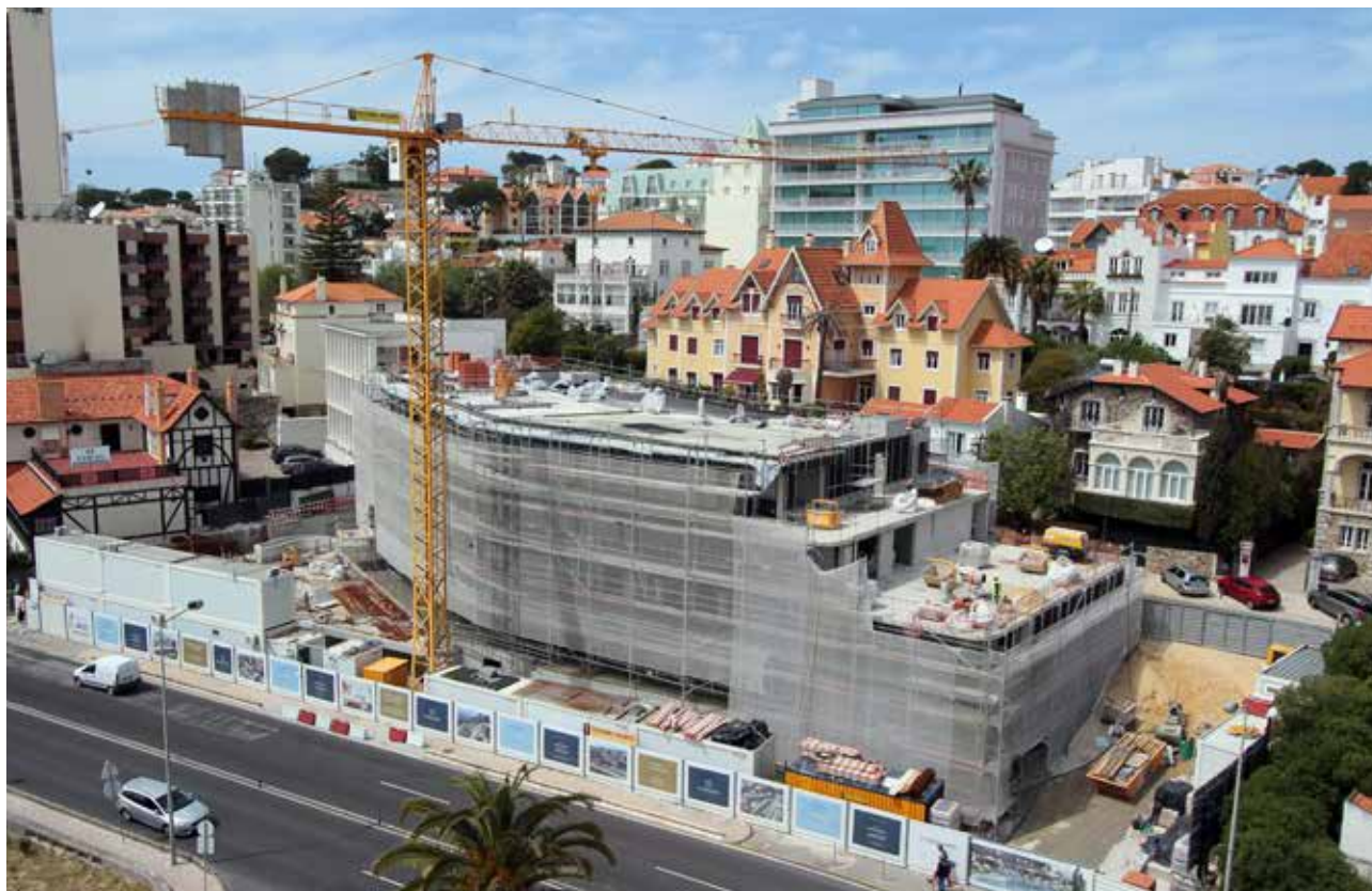
MONESTORIL - OCEAN RESIDENCE Monte Estoril - Portugal
