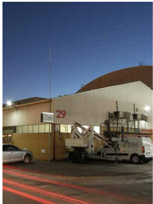
CAMPUS TAP - FM & Maintenance Lisboa - Portugal
