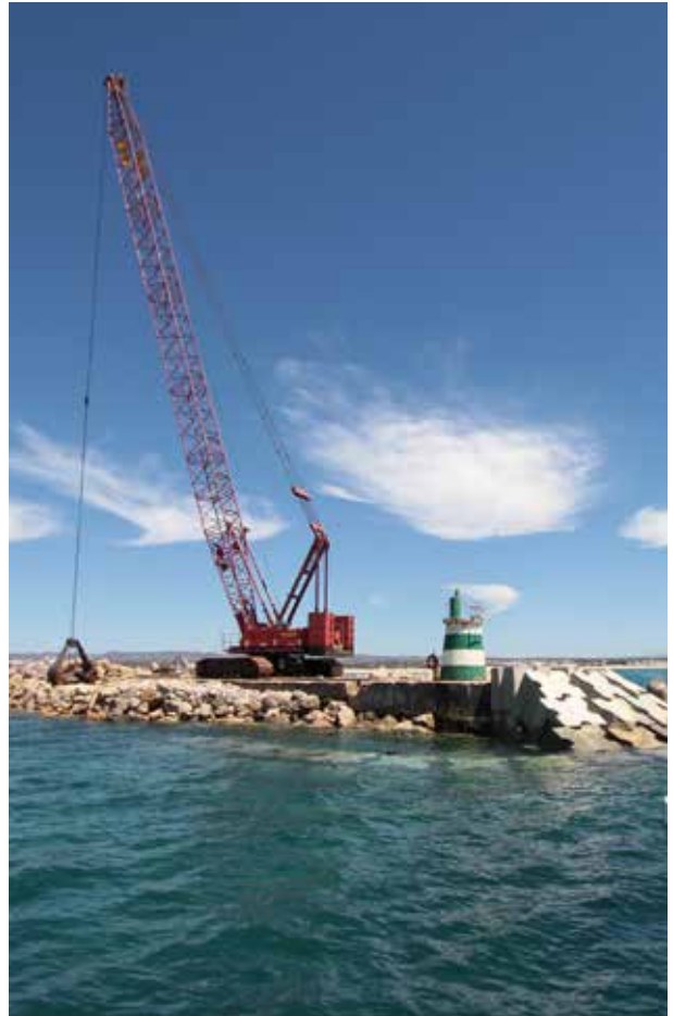
DGRNSS - REFURBISHMENT OF THE EASTERN BREAKWATER OF BARRA DE TAVIRA Portugal
