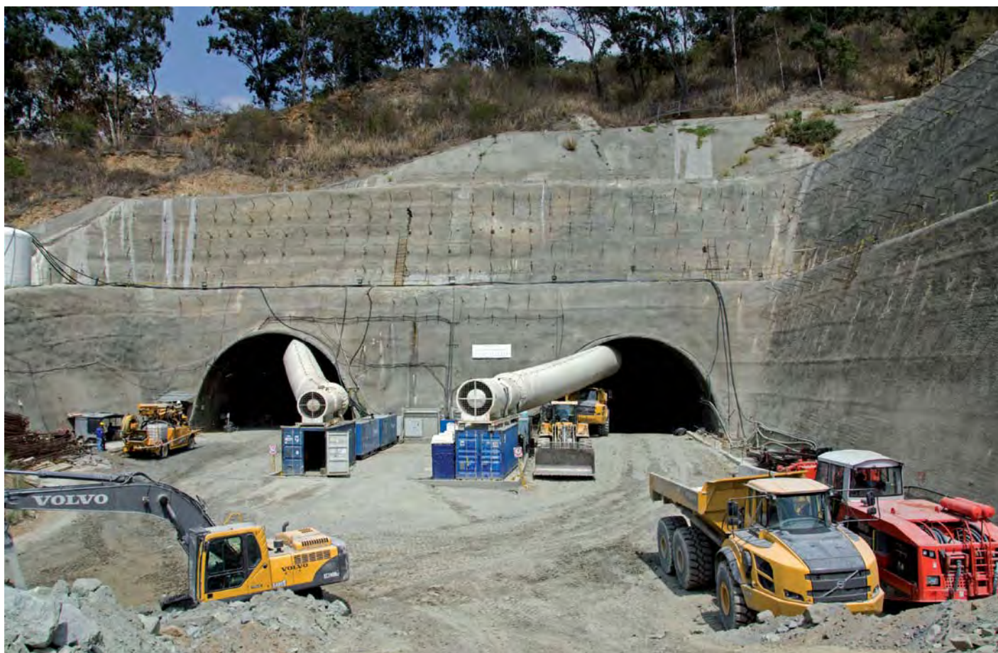
Consorcio Boyacá - La Guaira - Construction du tunnel de Baralt Caracas | Venezuela
